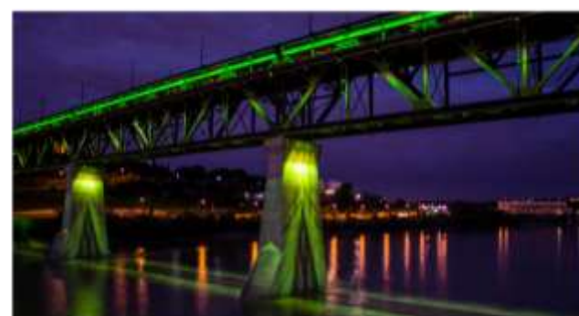
High-Level Bridge in Edmonton
