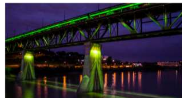
High-Level Bridge in Edmonton
